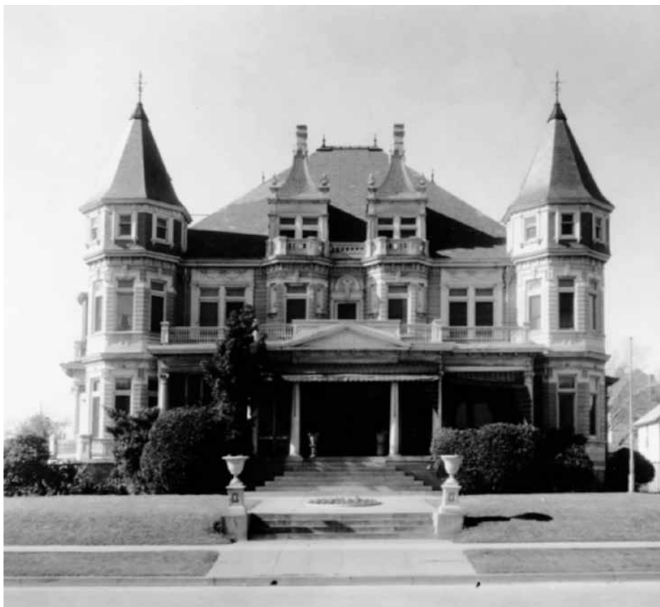
Levy Chateau, 2016 Main Street at Gray Avenue, built 1906, demolished 1938. Houston's Forgotten Heritage, p. 90.
