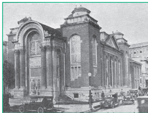
The second building, on the site of the first.
