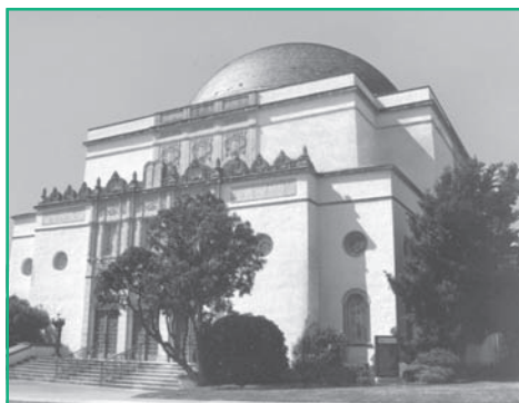
The third and current building.
