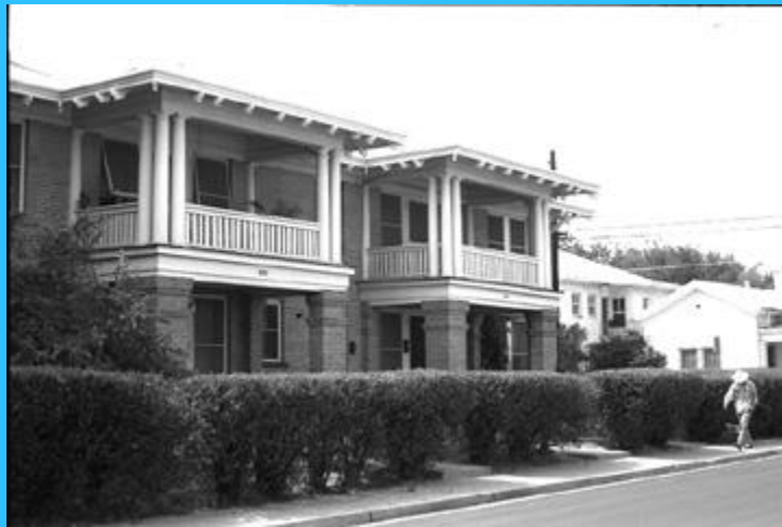
Apartment house typical of the neighborhood and the time.
